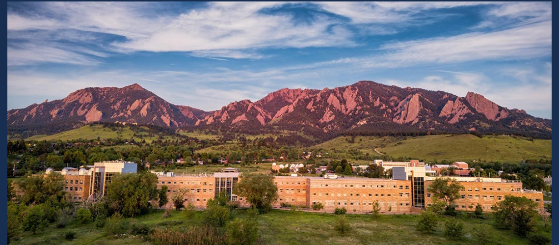
National Oceanic & Atmospheric Administration - Boulder, Colorado
